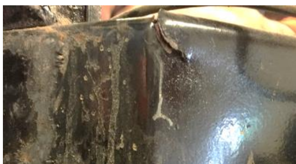
Figure 14. Cracking from sharp corners in frame
