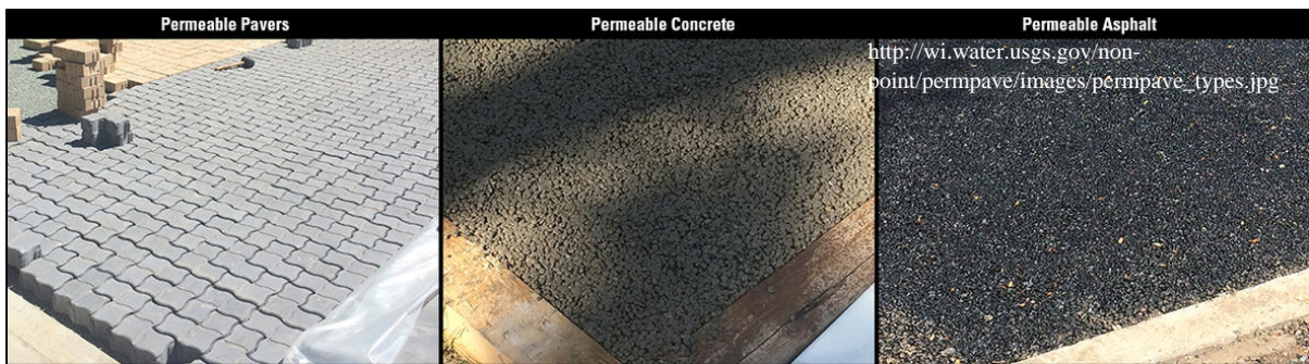
Figure 11. Different Types of Permeable Pavement
