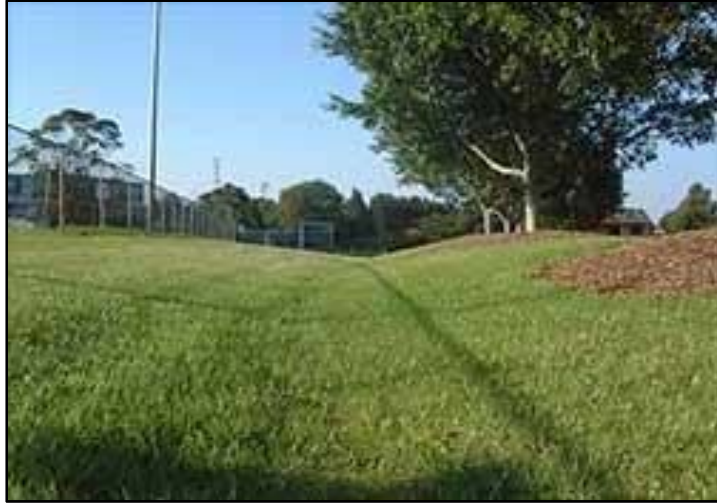
Figure 31. Simple Grass Swale
