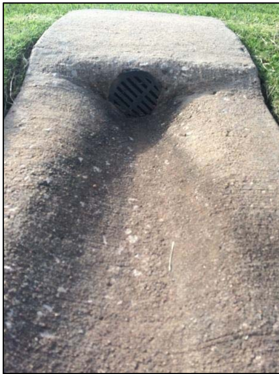
Figure 32. Undersized Drain
