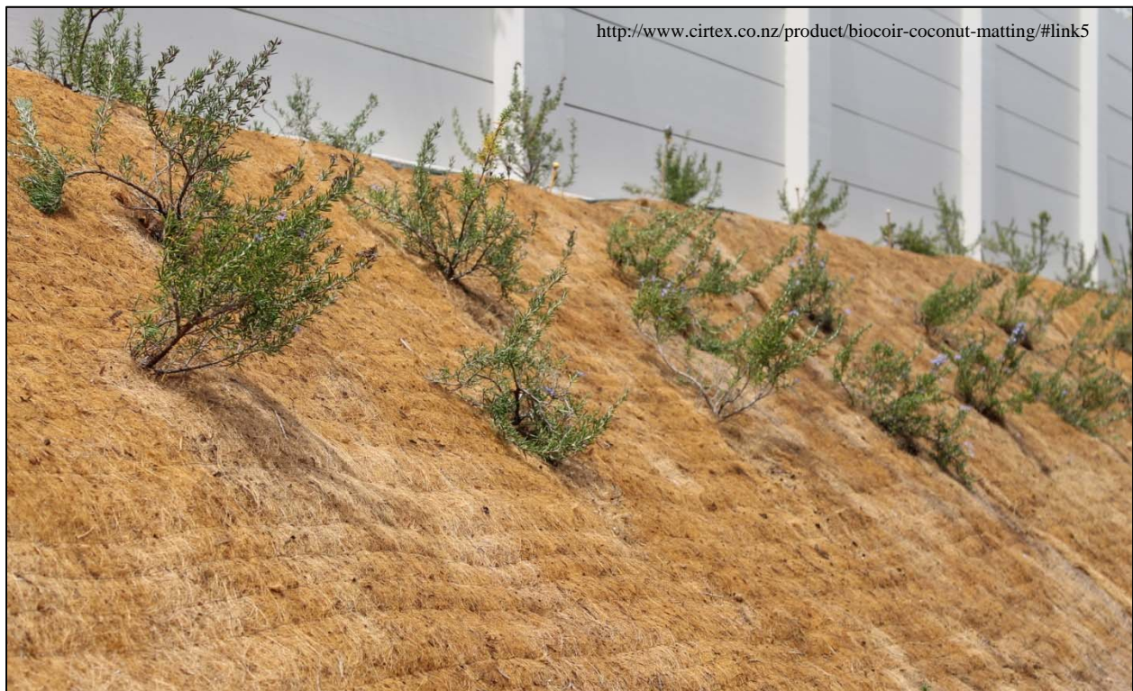
Figure 7. Combination of Live Stakes & Coconut Matting
