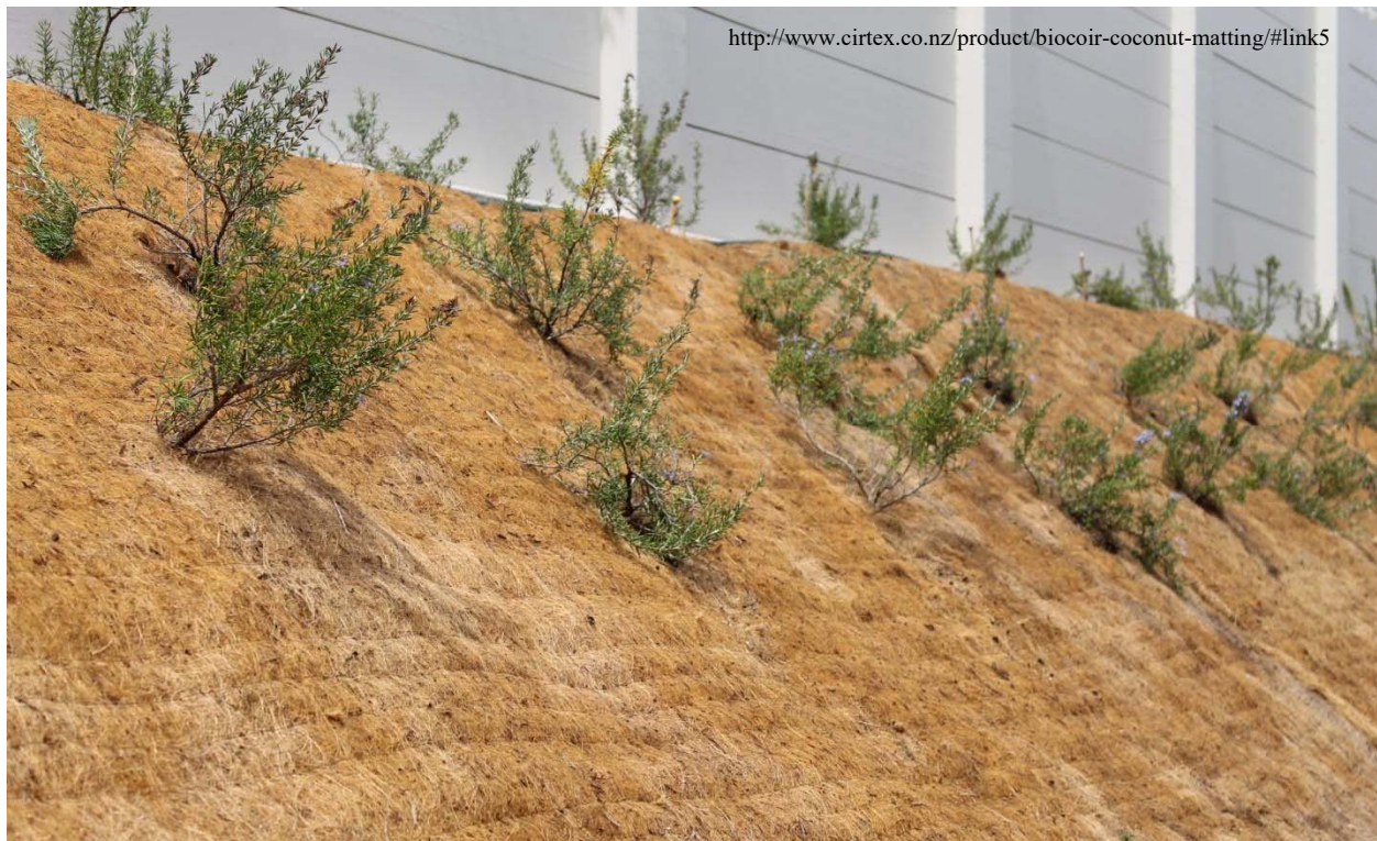
Figure 23. Combination of Live Stakes & Coconut Matting
