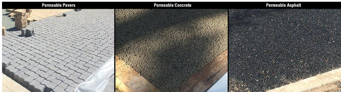
Figure 28. Different Types of Permeable Pavement
