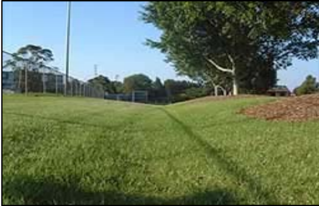
Figure 14. Simple Grass Swale
