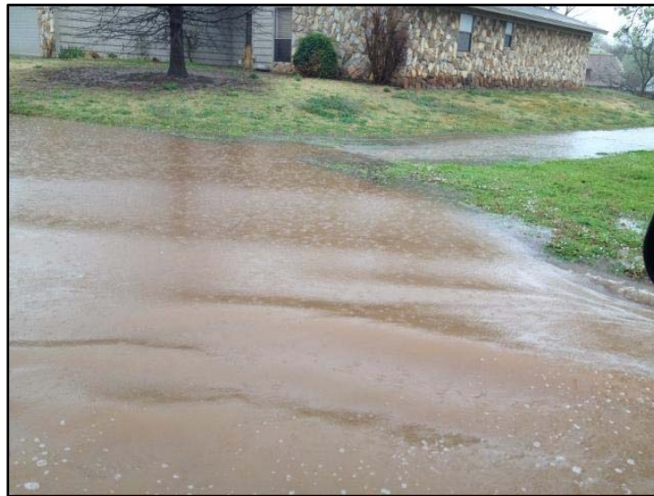
Figure 30. Ponding Observed at Park View Estates
