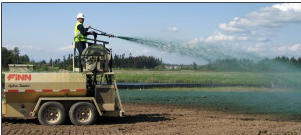
Figure 31: Example of hydroseeding (BAI Environmental Services)
