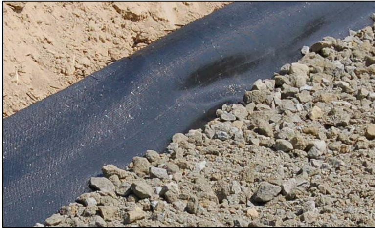
Figure 9: Woven textile fabric application (US Fabrics)
