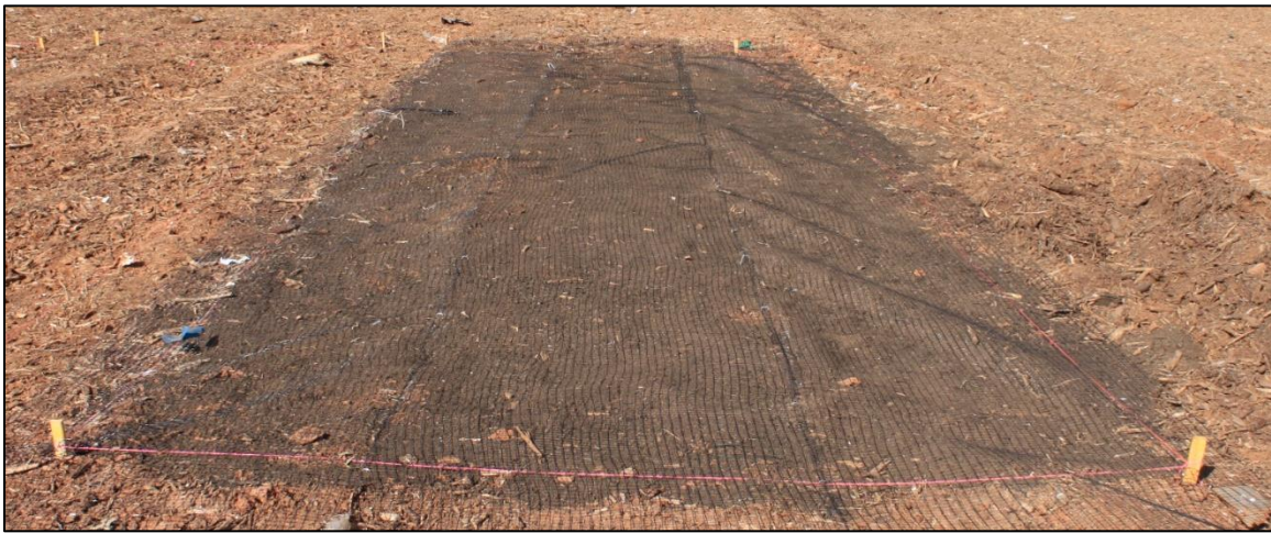
Figure 7: Image of installed compost blanket plot
