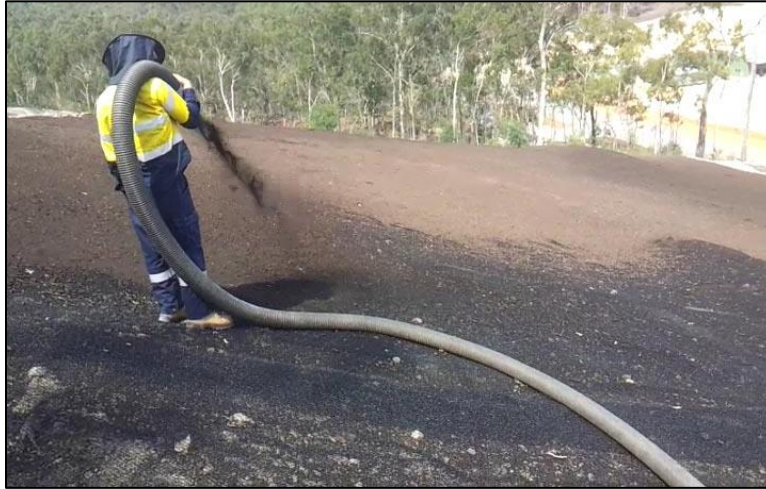
Figure 23: Example of compost blanket application (Integrate Erosion Control AU)
