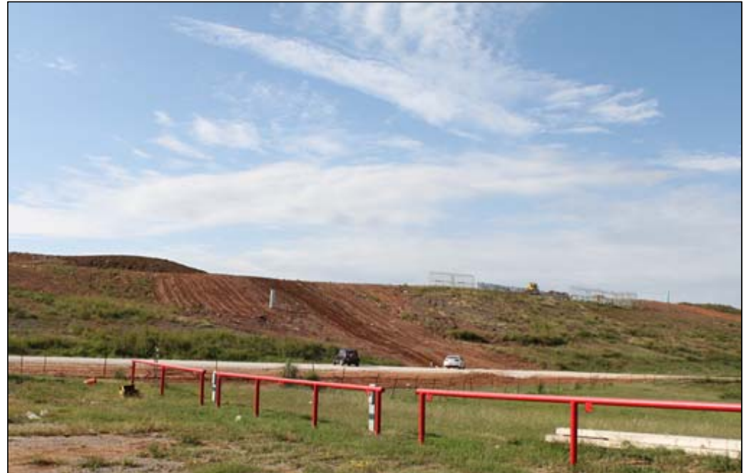
North-Facing Exterior Slope
