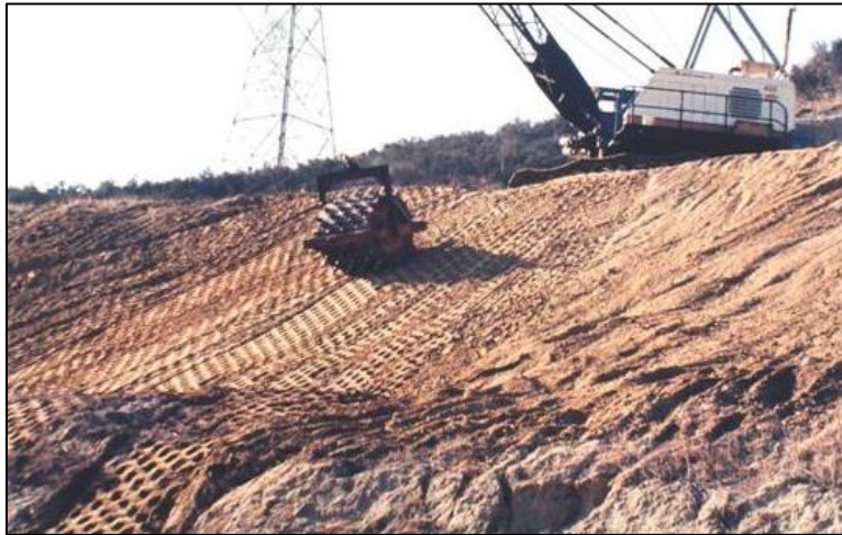
Figure 44: Example of imprinting a slope (The Imprinting Foundation)
