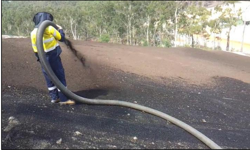
Figure 4: Example of compost blanket application (Integrate Erosion Control AU)
