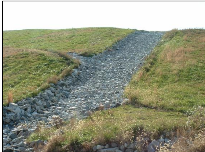
Figure 42: Example of riprap channel protection (Anne Arundel County, Maryland)
