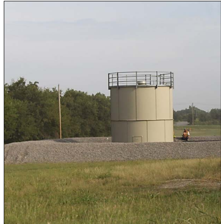
Enid landfill leachate collection tank
