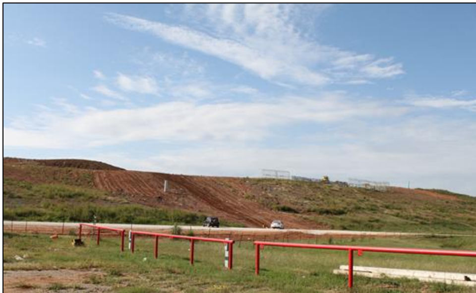
Figure 1: View of the North-facing slope of the Enid Landfill
