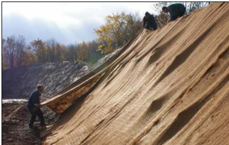
Figure 11: Coir textile fabric application (Bender)
