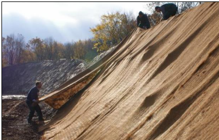
Figure 11: Coir textile fabric application (Bender)
