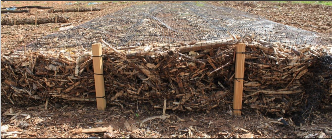
Figure 26: Image of homemade woodchip berm
