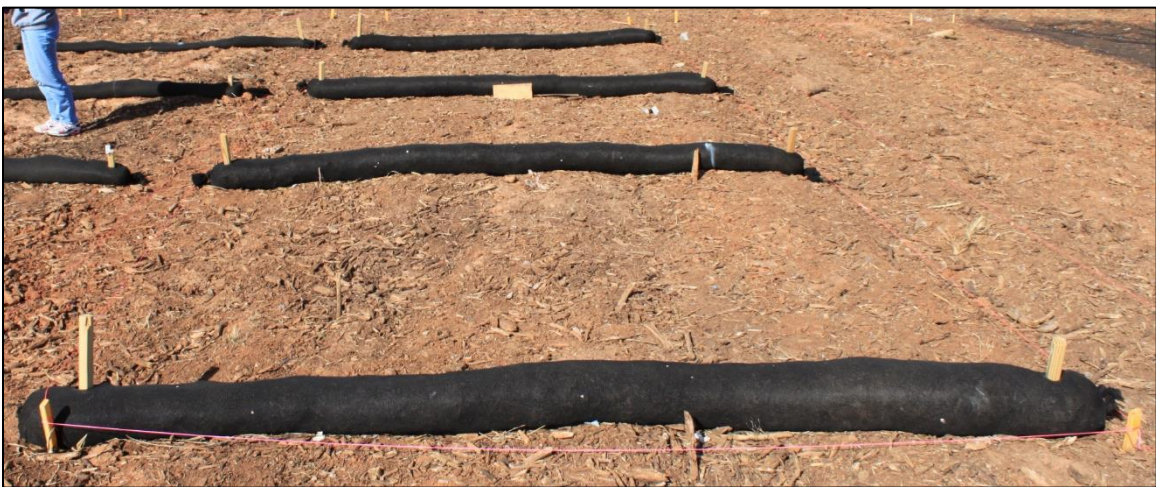
Figure 10: Image of installed manufactured compost sock plot
