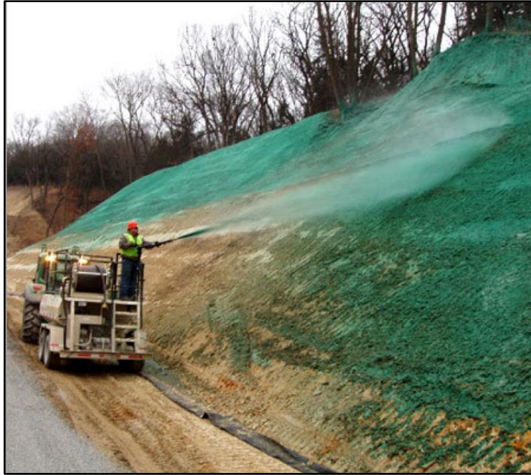
Figure 3: Example of hydroseeding application
