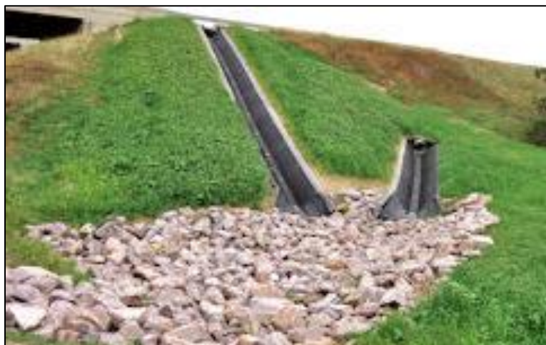
Figure 43: Example of water channeling (Stormwater Solutions)
