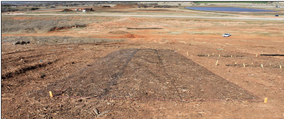
Figure 15: Image of installed biosolids and woodchips plot
