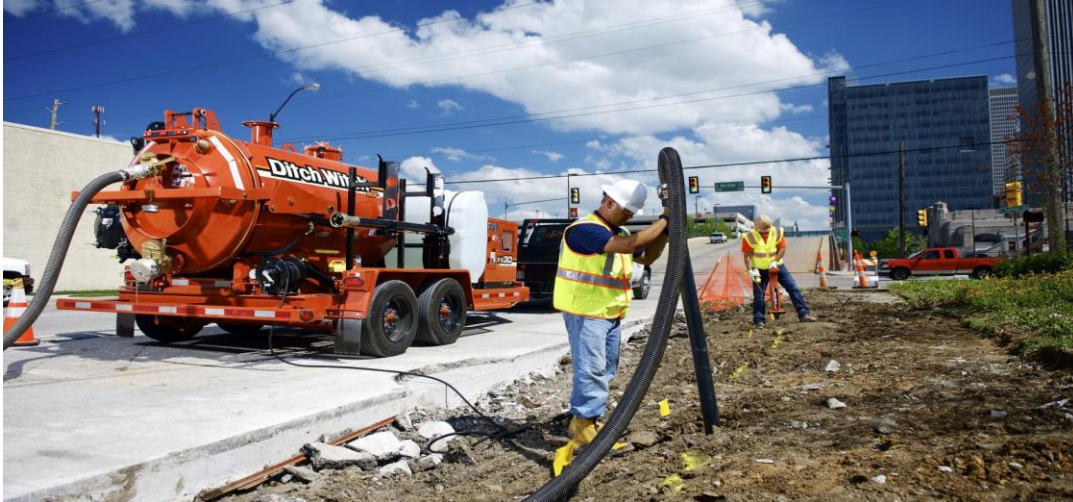
Figure 2. FX-30 vacuum excavator in the field.
