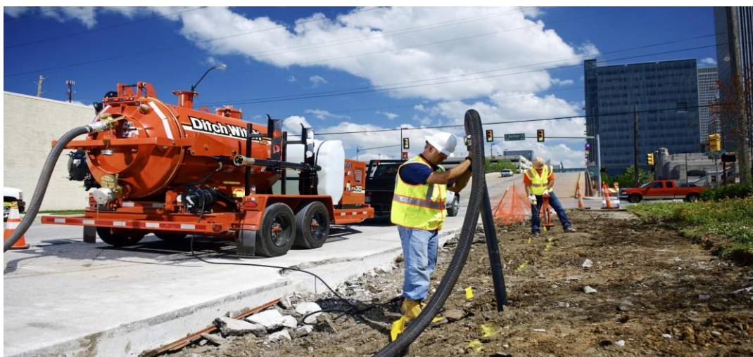
Figure 1. FX-30 vacuum excavator in the field.
