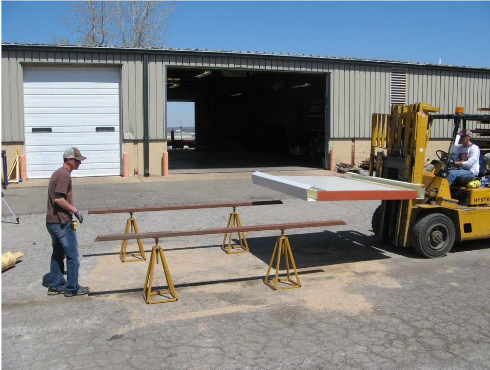
Figure 16: Loading the Test Wall on Simply Supported Beams
