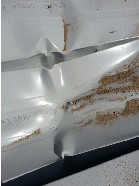
Figure 39: Indentation from 2x4
