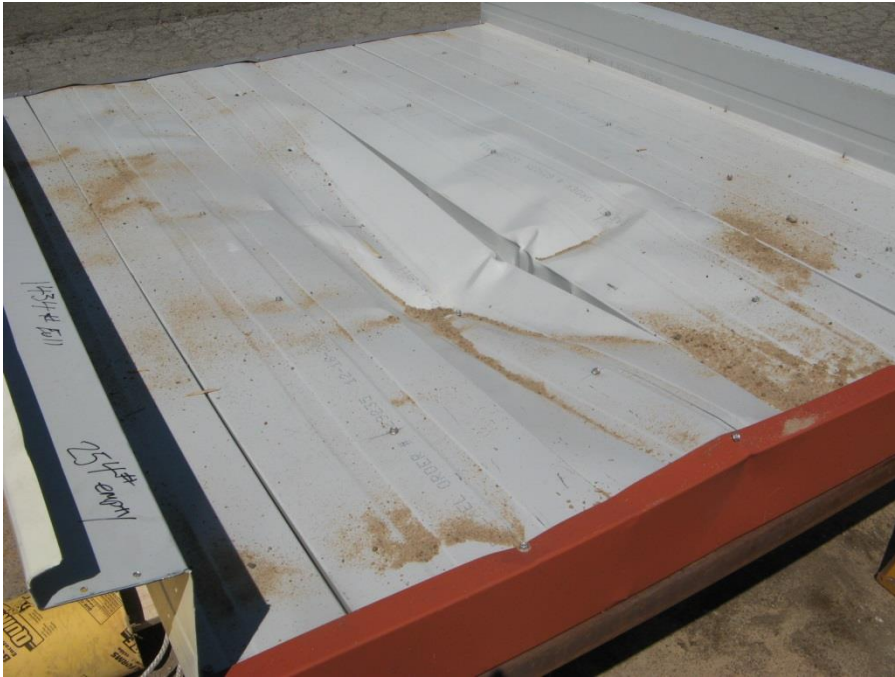
Figure 36: Damage from Test 2 and C-channel Deformations
