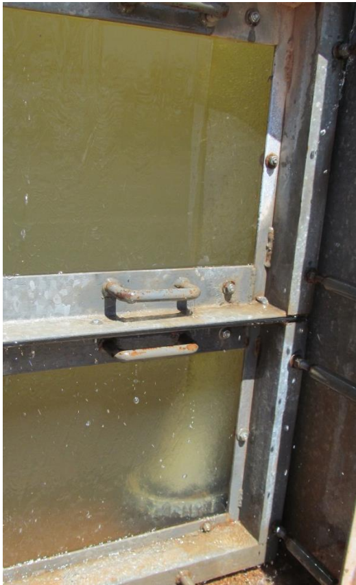
Figure 11: View of the diffuser through the window.
