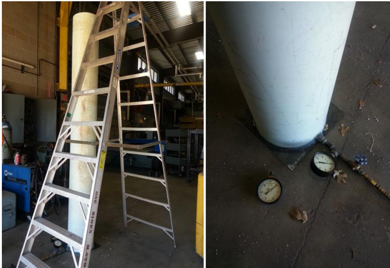
Figure 9: Testing of compressor requirements.
