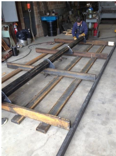
Figure 16- Laying out the center shaft into table
