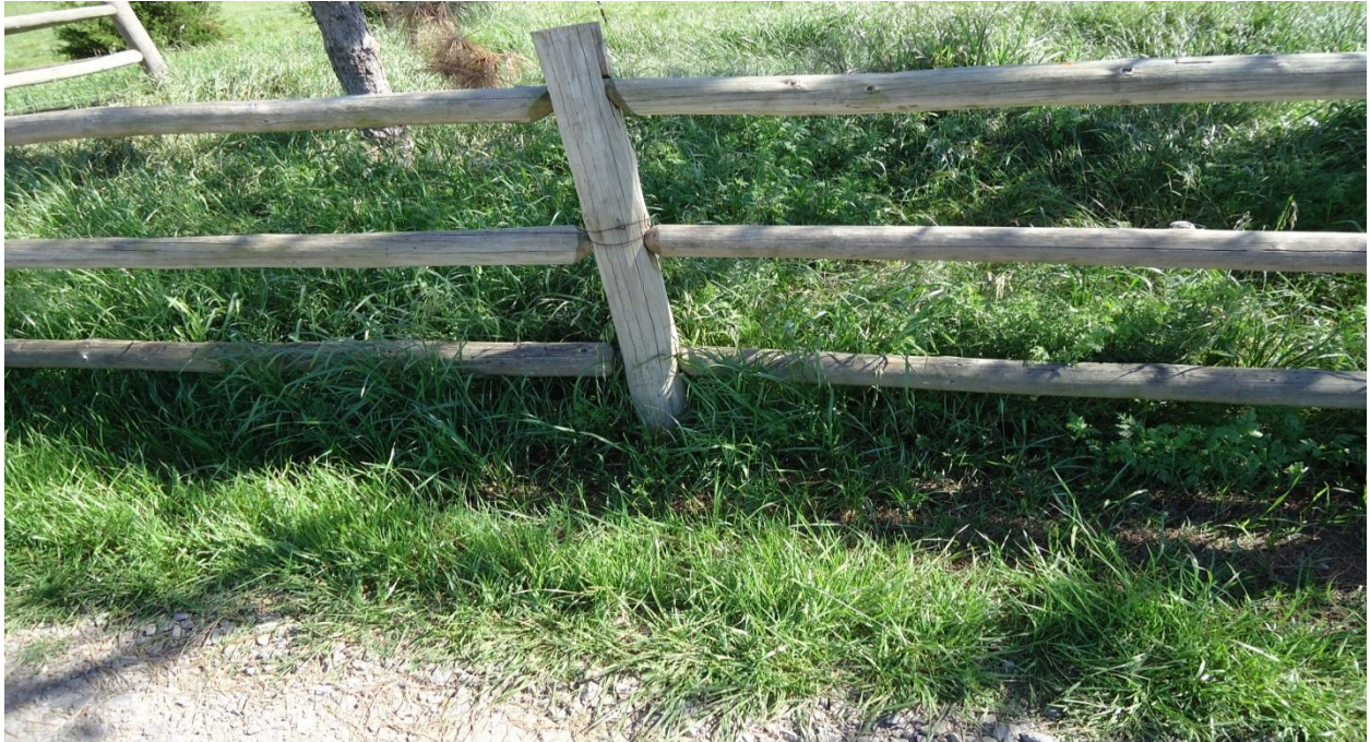
Figure 20 - Another picture material for cutting.
