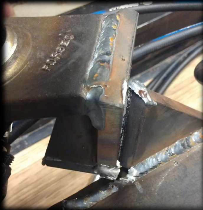
Cylinder Mount (Bad Weld)
