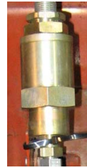
Figure 11: Check Valve
