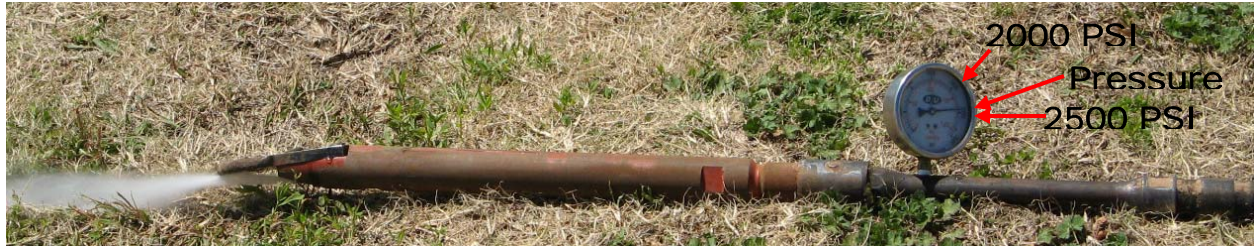
Figure 30: Full Drill String Pressure Reading
