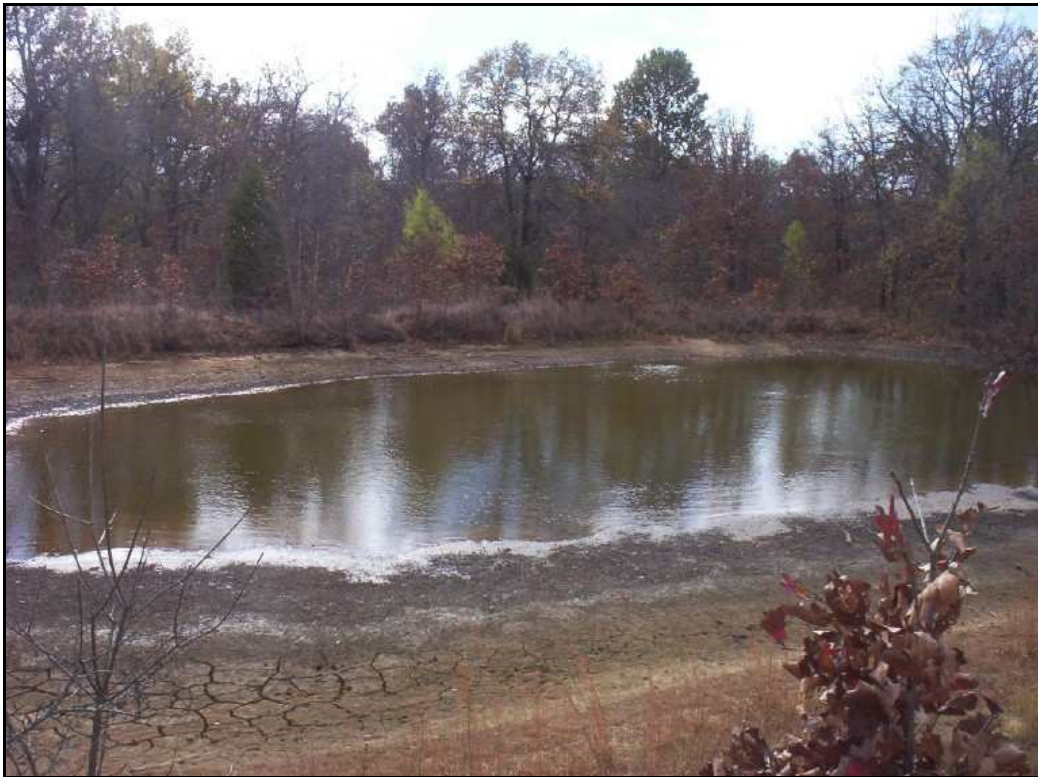
Figure 18. Current wastewater lagoon conditions
