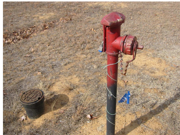
Figure 4: Current fire protection standpipe.
