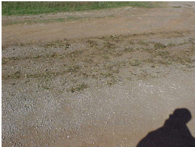
Fig. 4 In the right picture the lack of consistency in the application of the sprigs is easily seen by the streaking and clumping.
